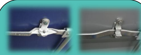
Door handle and retainer catch with security holes (left) and with normal catch (right). Repair should be like for like.
